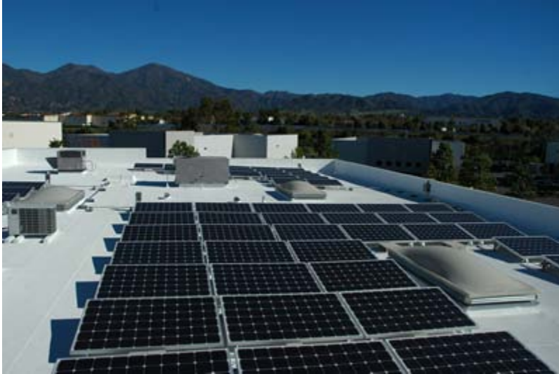
Installation of solar photovoltaic panels on a cool roof in Rancho Santa Margarita, California. Photo courtesy of Coat 'N' Cool.
